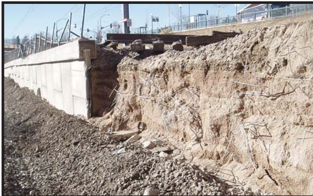
Dismantled MSE Wall, Jan 19
