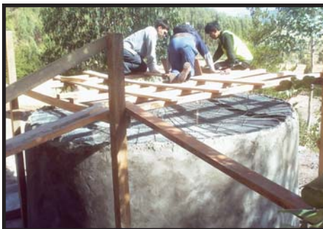
Work underway on ferro-cement chlorination vault in Peru
