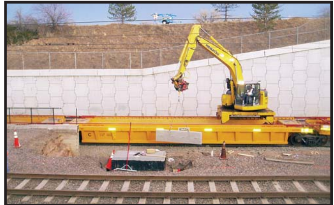
Reconstruction underway, Jan 20
