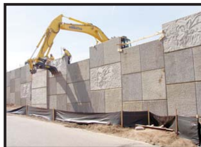
Construction now underway on 'FasTracks'
